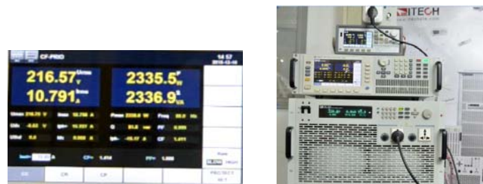
Picture 6 Screenshot of over current protection point
